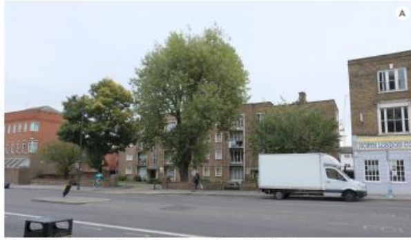
View of Reynardson Court from Tottenham High Road
