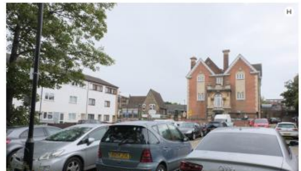
View of Holy Trinity Primary School from site
